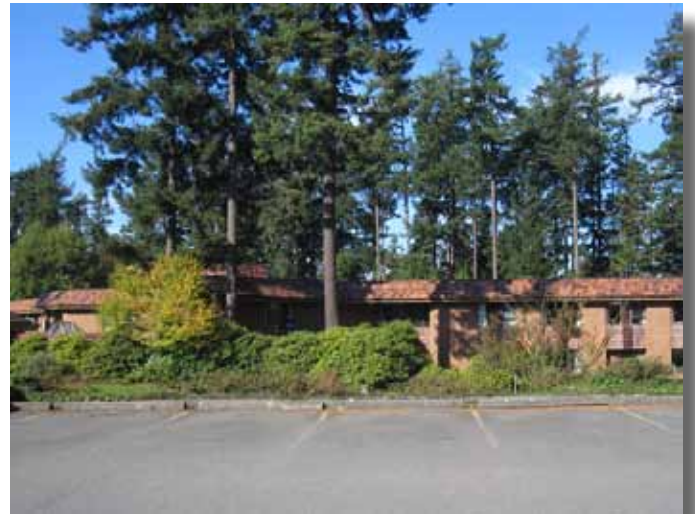
Existing building at Queenswood.
